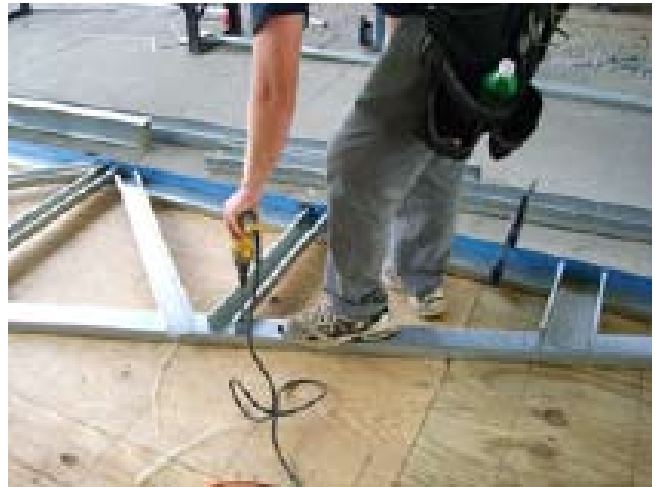
Step 3. Webs are screwed to the top and bottom chords.
