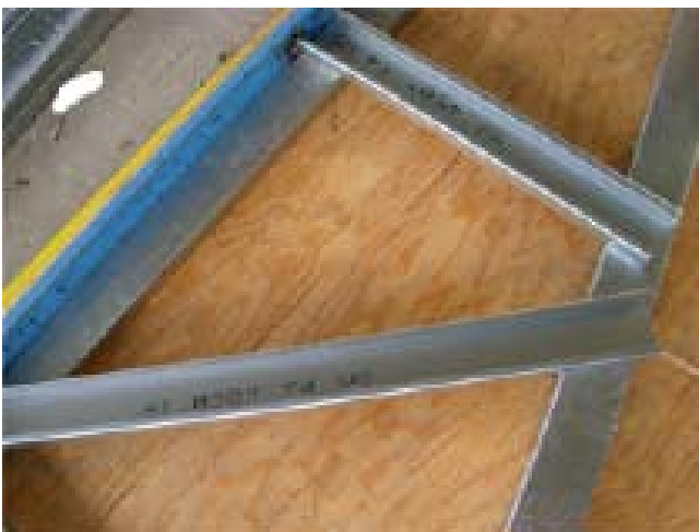
Step 2. Machine-labeled stock is placed in the jig
