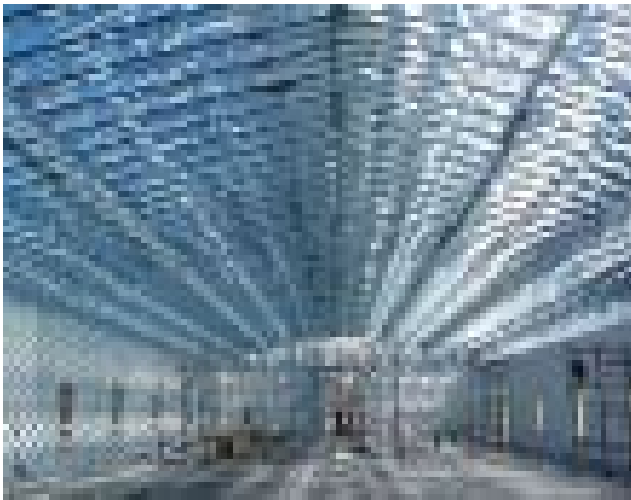
Scissor Truss (shown) provide a dramatic ceiling effect. This truss type will exert lateral forces on walls if not installed with a fixed and slide end.
