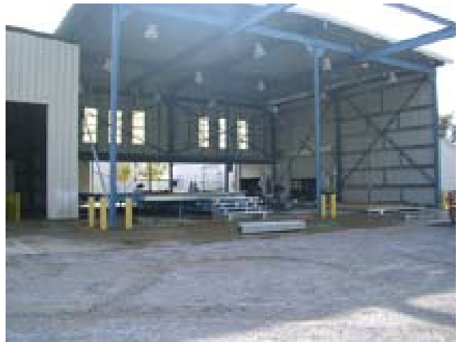
Step 4. Trusses are loaded onto trucks directly from the assembly stations. This assembly station, located in Freeport, FL has a built in crane/boom assembly to place trusses directly onto waiting trucks.
